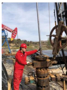
a The instrument goes into the wellhead
